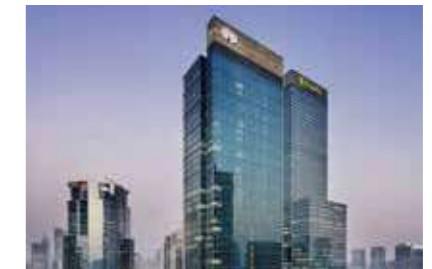
JING AN KERRY CENTRE Shanghai
